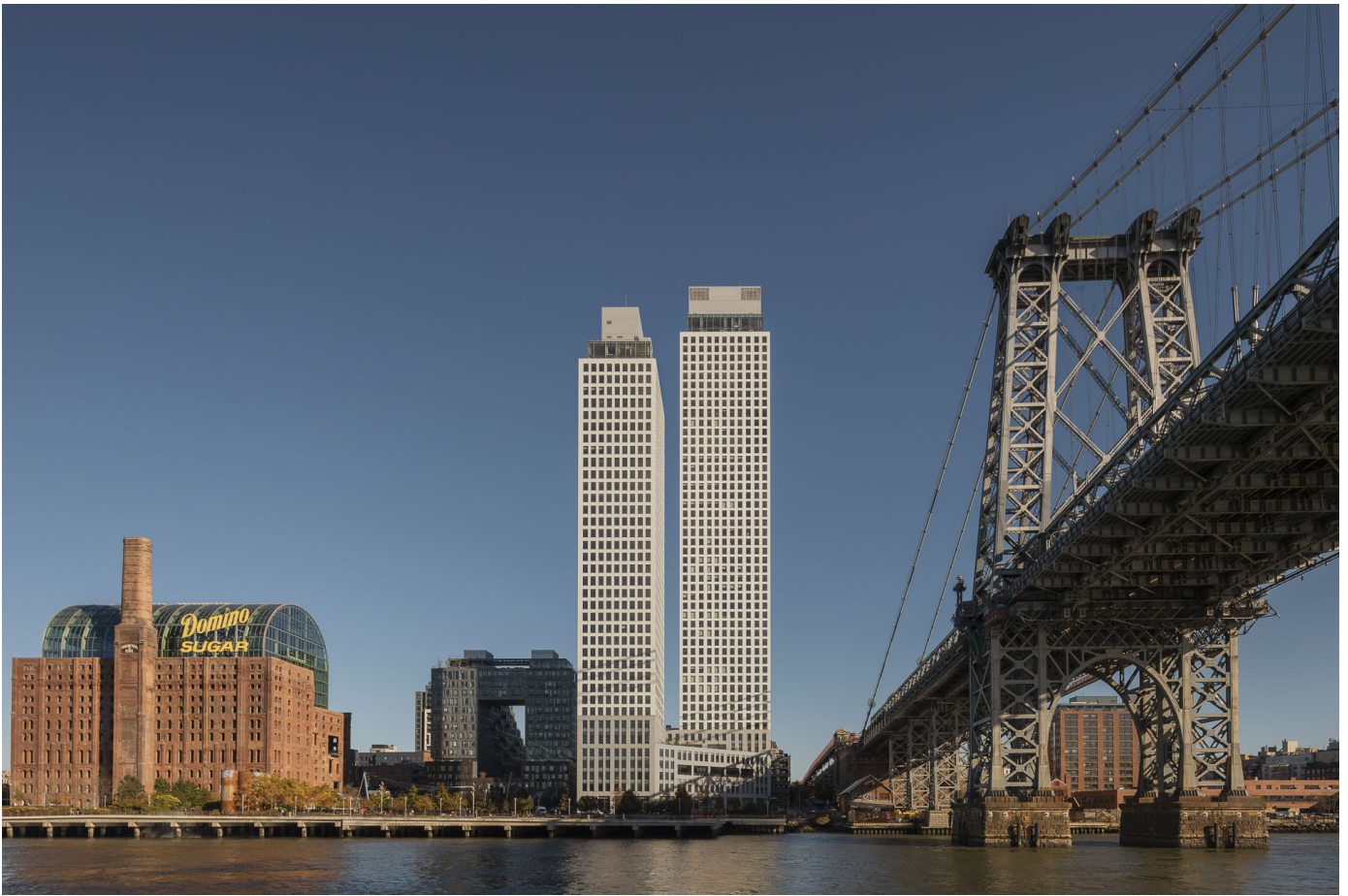
One Domino in Williamsburg: The pearl-like, porcelain-clad facades of the two towers change depending on the light, the time of day and the weather. © Ivane Katamashvili
