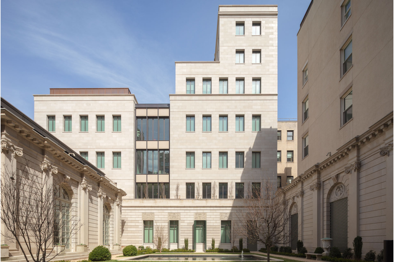
In the extension to the Frick Collection in New York, Selldorf draws on the material palette of the historic buildings and also uses Indiana limestone in a rusticated finish. © Nicholas Venezia
