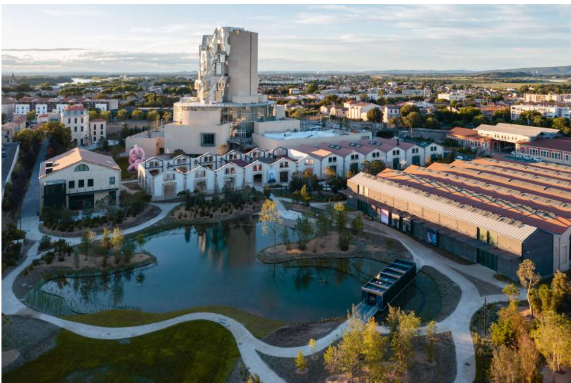
Luma Foundation, Arles, France
