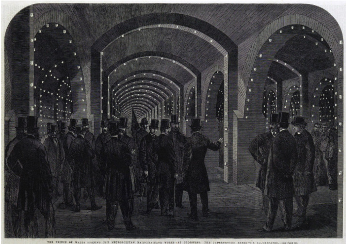
THE PRINCE OF WALES OPENING THE METROPOLITAN MAIN-DRAINAGE WORKS -AT CROSSNESS: THE UNDERGROUND RESERVOIR ILLUMINATED.—MR. PAGE DEL.
