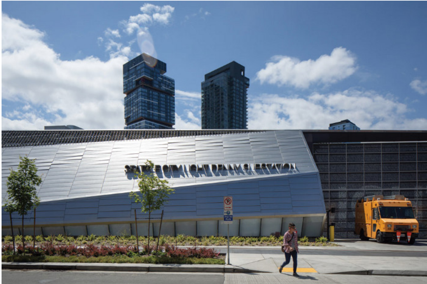
The glass and steel Denny Substation by NBBJ Design provides power to the evolving South Lake Union neighbourhood in Seattle. Image credit: Sean Airhart
