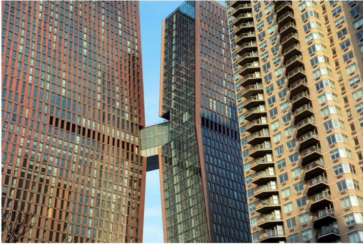
At center and left, SHoP's American Copper Buildings. The bridge between the two towers contains a swimming pool. Photo: Bo Zaunders/Getty Images
