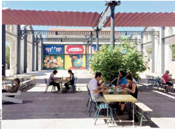
10, 11 gli spazi espositivi con le strutture originali: pareti portanti in muratura, colonne in ghisa e capriate in acciaio exhibition spaces with the original structures: load- bearing masonry walls, cast-iron columns and steel trusses
