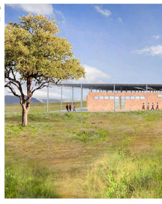
The corrugated metal roof at 6.6m high is designed with an aspirational scale to reflect the promise of the students. A covered assembly space is left open to the local road, marking the entrance and welcoming students. In addition to serving as the school lunch hall, it will be a resource for local civic gatherings.
