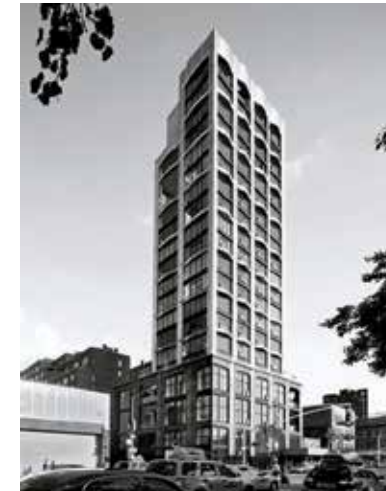
The exclusive residential tower at 200 11th Avenue has a 16-storey tower perched on a three-storey plinth that's clad in terracotta to suit the neighbourhood.
